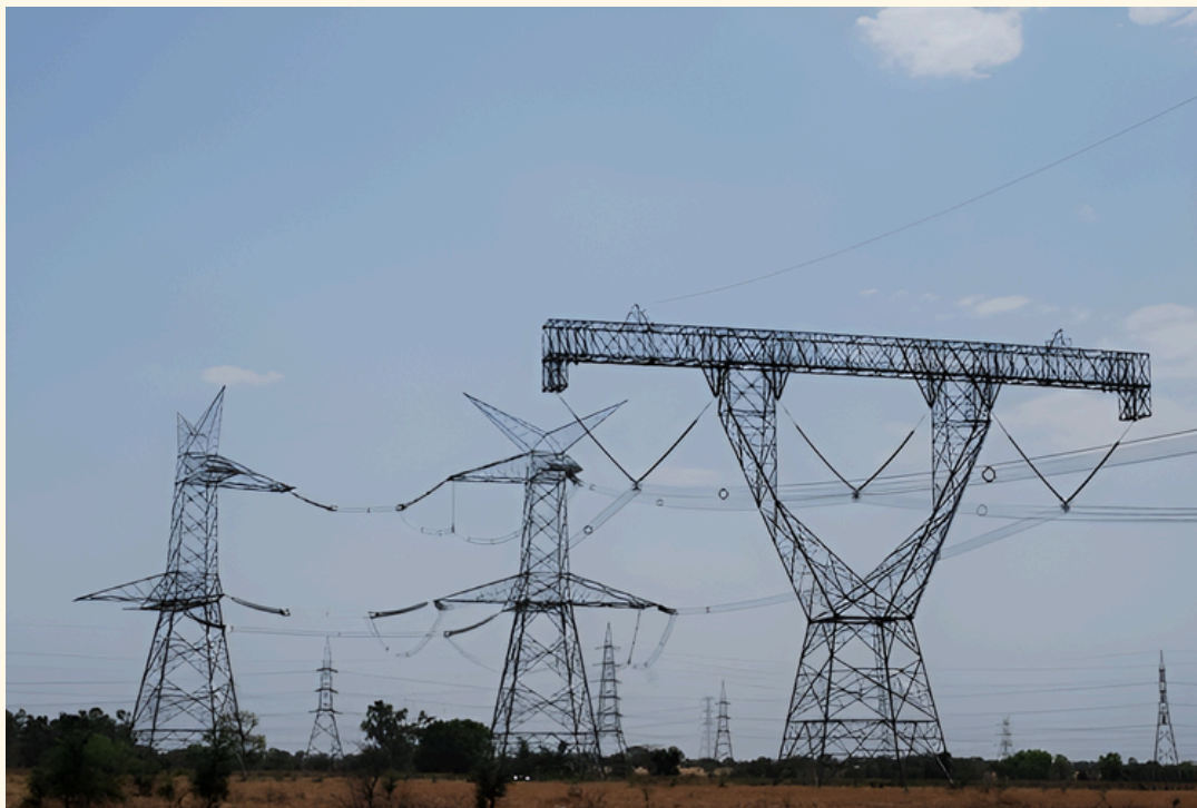
India's 1200 kV Transmission Line at Bina Substation
